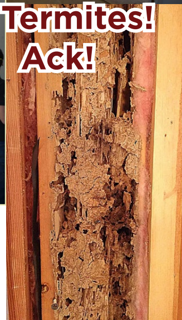
Extensive termite damage found around main entrance.
